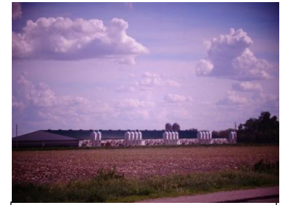
Example of an Animal Confinement Building
