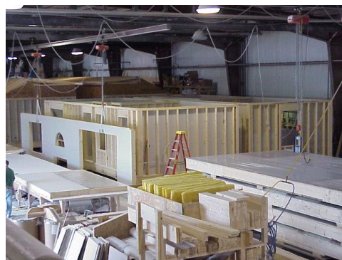
Example of a Dwelling, Manufactured Home Source: http://transportablehomesspecialist.com/
